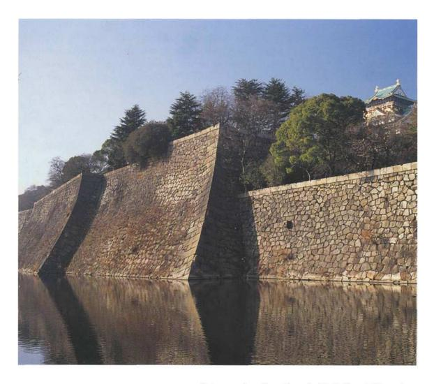
This view of Osaka's walls shows how a long wall could be concertinaed into a design known as byobu (folding screen). This allowed for the important element of heavy flanking fire from hundreds of arquebuses. The huge stone walls seem to dwarf the great keep of Osaka that appears in the distance.
