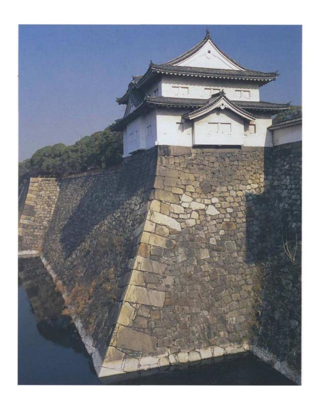
A corner tower of Osaka castle shows the angle of the stone-clad base. The edges are neatly arranged using huge dressed stones.
